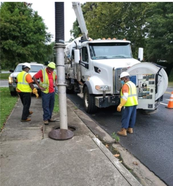
Crews using seen here are using a Vac truck to remove debris from one of nine catch basins. September 2020
