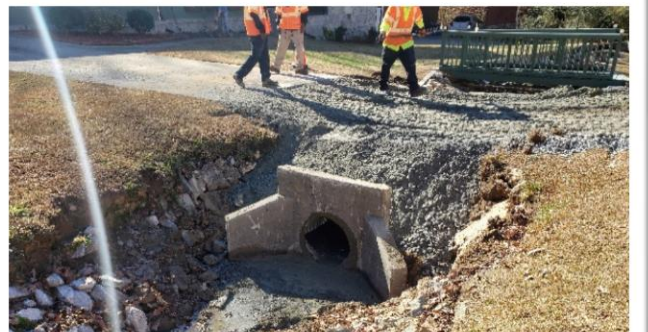
Restoration to bank after new installation of CMP September 2020
