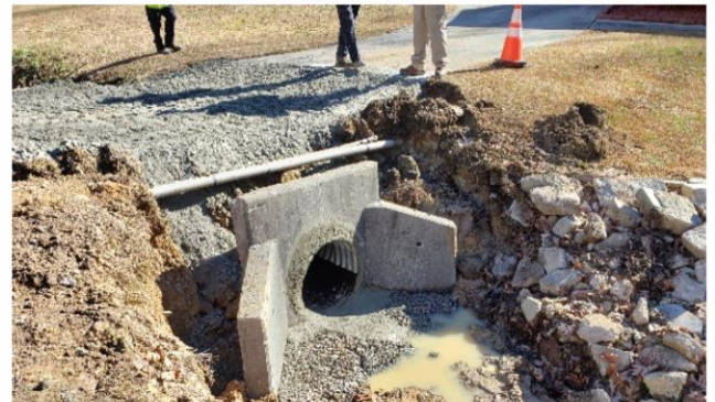
Corrugated Metal Piping (CMP) being installed at resident's home along Marcus Nyah – September 2020
